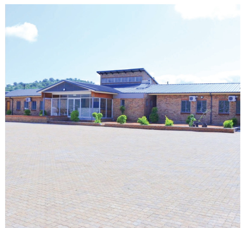
The new traditional council offices at Ga-Manoke Village are expected to restore dignity and strengthen traditional governance.
